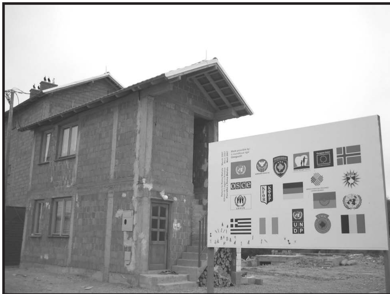
New housing in the Mitrovica Romani Mahalla, built by Norwegian Church Aid and Danish Refugee Council with international funding. The quality of the houses built and civil planning of the area leave much to be desired.
