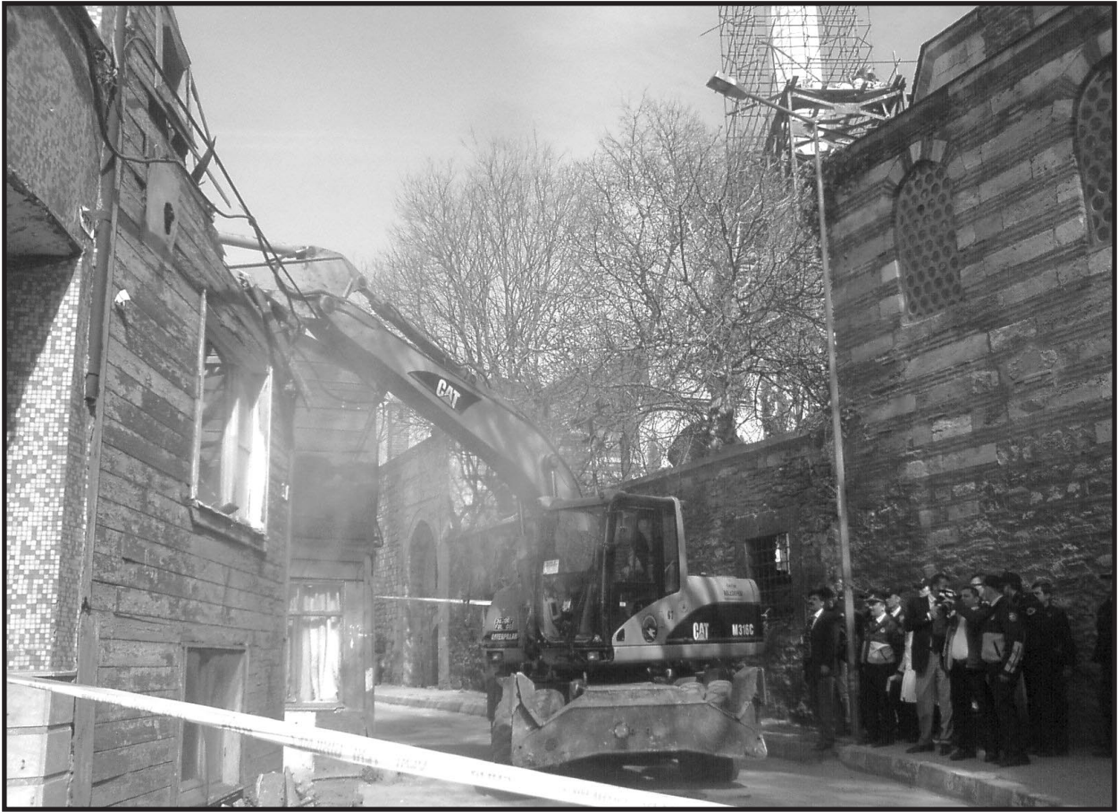
The Urban Renovation Project of Sulukule is under legal scrutiny by a Turkish court due to a case submitted with the support of the ERRC. Despite this fact, demolitions continue in Sulukule. In mid-March 2008, excavators of the Municipality were again at work, this time razing a total of seven houses.
